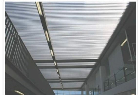
Upgrade Sydney Airport Terminal 1 Car Park
